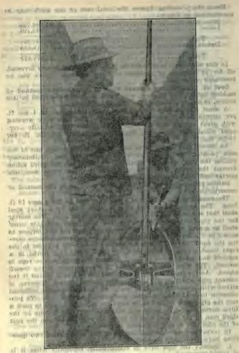
Fig. 30.—Ransome Cement Pipe Mold in Trench.
